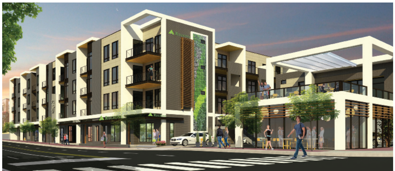
GBT's Diversified Division is developing Village 21 at Regents Park in the upscale Hillsboro neighborhood of Nashville. The mixed-use development has 101 multifamily units on top of retail space.
