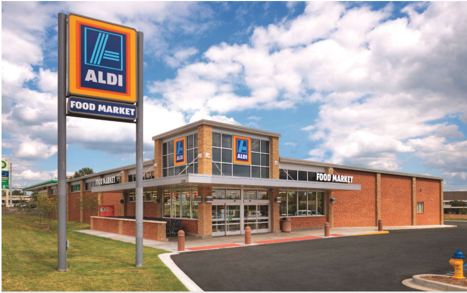
Morgan Construction will build its 100th and 101st Aldi stores in Conway, S.C. Aldi recently announced a $1.6 billion remodeling plan to enhance 1,300 stores.
